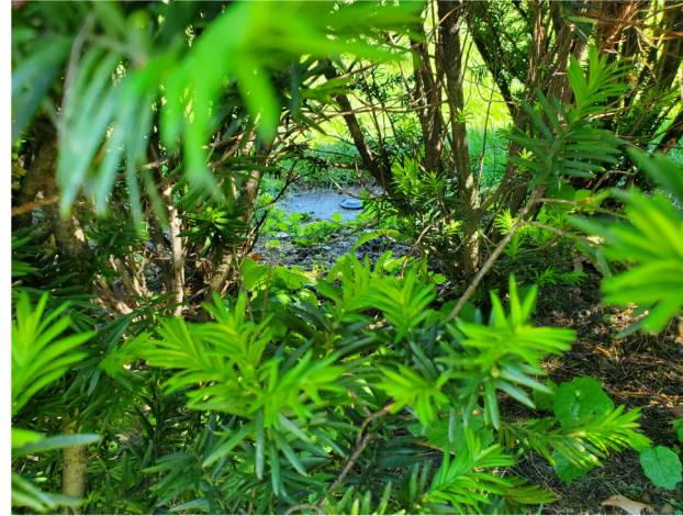
(Manhole seen through bush)
