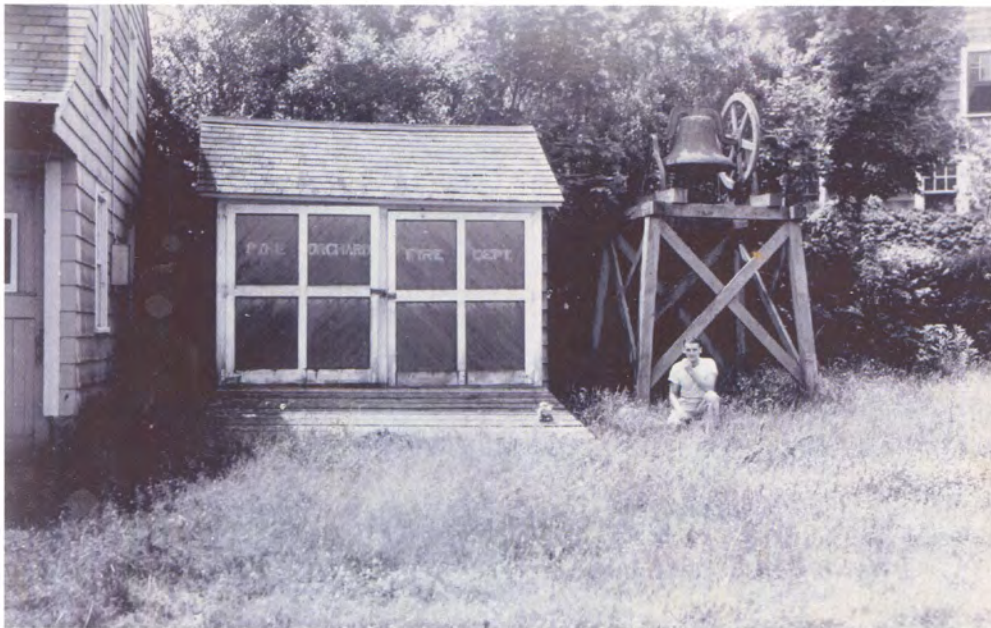
Fire alarm bell on the side of fire house
