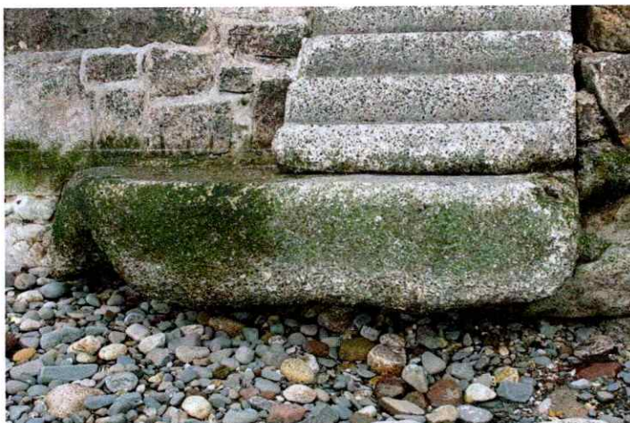
Existing site conditions as shown in permit application 202303146-COP
